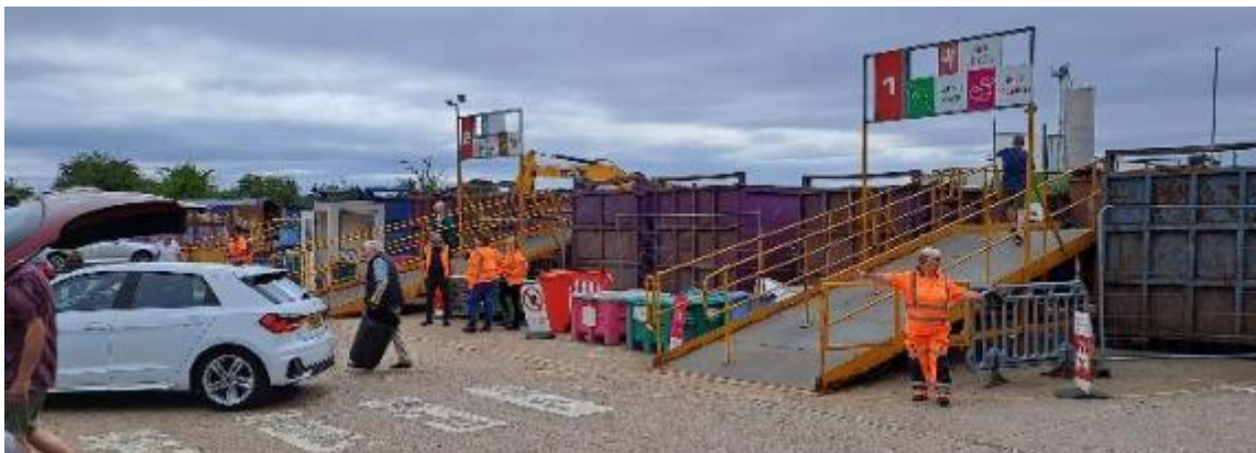
Figure 1.11 Parking and Access Ramps at the Wellingborough HWRC
